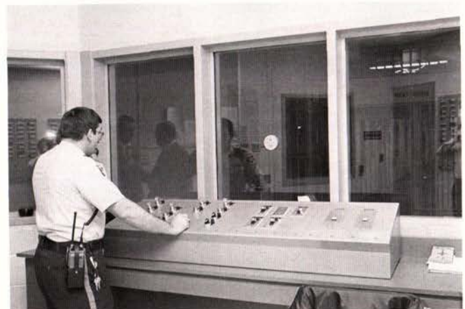
Elevators are operated by remote control from the corrections officer's station on each floor.
